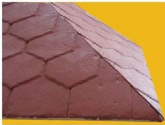
Picture 1: Install shingles on to the sides of the hip as shown above.
