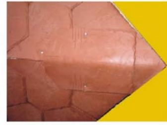
Picture 3: Install the next shingle as shown above. Additional nails may be used to firmly secure shingles. Repeat this step until you reach the top.
